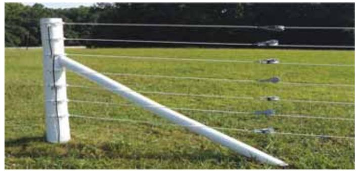
Loop is made from high tensile wire covered with a polymer blend, so no insulators are needed.
