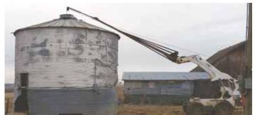
He made a 16-ft. long boom for his skid loader and used it to lift bin's roof and top ring of panels.
