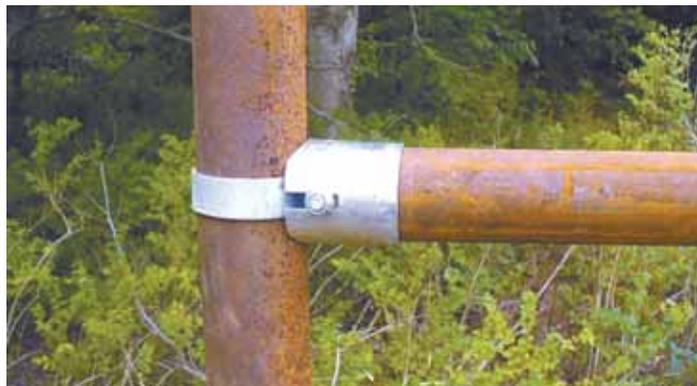
Pipe connector kit includes a band that clamps onto a 2 7/8-in. pipe post, and a double-slotted sleeve that slides over a 2 3/8-in. cross pipe. A carriage bolt runs through band.
