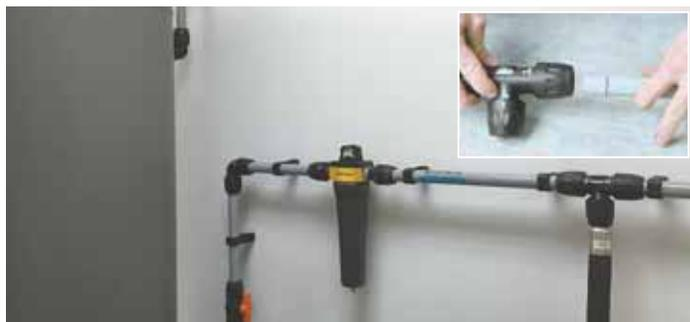
DanAm compressed air piping system goes together with “push to connect” fittings. The modular design uses reinforced nylon couplers (inset) to connect runs of pipe together, making it easy to assemble, change and expand.
