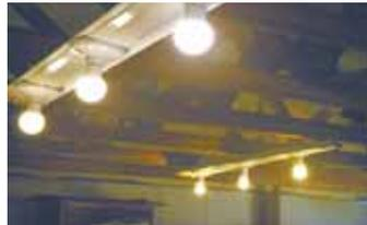
**Bill Halstead, Lacey, Mich. (269 758-3232):** "I couldn't justify spending money for new LED light fixtures in my shop, so I came up with a cheap way to install LED bulbs. I removed the ballast from my fluorescent lights and used the existing wiring to install the bulbs. My only cost was for new LED bulb sockets which I bought for \$1.46 apiece."
