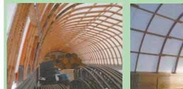
Silver Stream makes hoop barns with either steel or wood hoops. The advantage of wood is that it's easier to insulate and it can be tinned over at any time, if desired.
