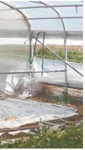
Rollers at the base of sidewalls roll back and forth on rails.
