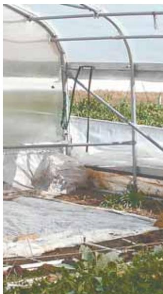
Rollers at the base of sidewalls roll back and forth on rails.
