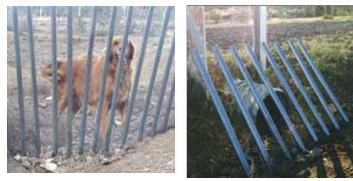
"It keeps trash from catching on wire fencing and culverts," says Joe Pacheco about his "pipe fence" kit. It consists of a reusable metal template that helps drive pipes that work with the flow of water.
