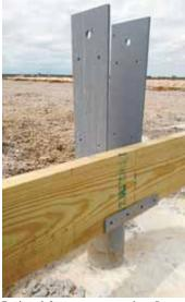
Designed for new construction, Strong Way Column consists of a galvanized steel frame that's backfilled with concrete. It comes with a built-in grade board bracket.
