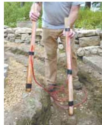
Ruen used plastic tubing and 2 yardsticks to make a water level for maintaining grade, while using a rototiller to dig a 190-ft. long drainage ditch around his house.
