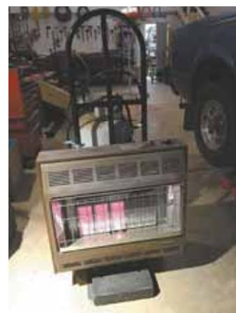
**Wall-mount, non-vent propane residential heater straps onto 2-wheeler where it can be easily moved anywhere in Payne's shop.**
