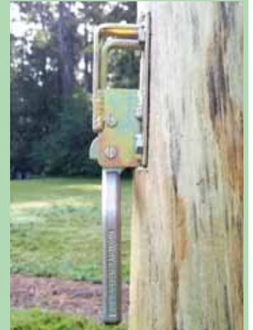
“Drop” gate latch consists of an upper catch latch and a hinged, 2-pronged fork. Pulling the catch latch up drops the fork, allowing gate to swing in either direction.
