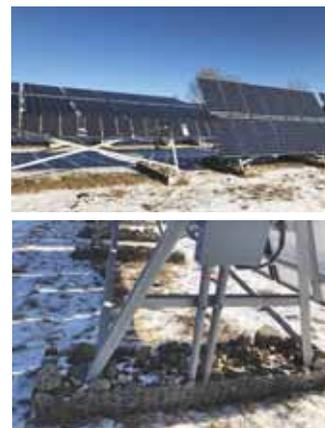
Solar panel racking kit provides an inexpensive way to anchor A-frame steel stands that support panels set up in series. Each stand is anchored by a rectangular rock-filled base made from expanded steel mesh.
