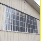
We have a large barn with a bi-fold door It has always been quite dark inside the barn. We decided to remove part of the metal sheeting which covered the door and replaced it with clear corrugated plastic. Now the sun shines directly through the plastic and we have a well-lit barn using free light. The cost was minor. Of course, we live in California - not sure how this would work in an extremely cold area. (Ron Ziegler, ph 805 344-6400)
