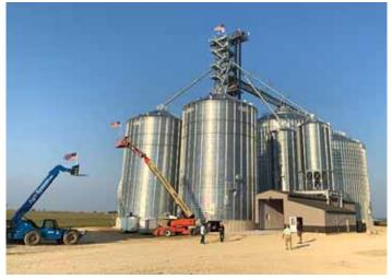
Their new grain handling system consists of 3 grain legs in a single tower, two 500,000 bu. bins, two 100,000 bu. bins, two wet grain hopper bins, a 10,000 bu. loadout, a double pit dump, and a certified scale with a control center.
