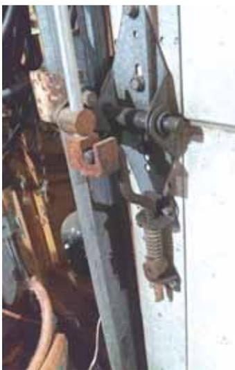
**By closing the door, a spring-loaded hook latches into a slot. As wind moves the door, the latching spring will pivot the latches tighter, holding the door tight to eliminate gaps.**
