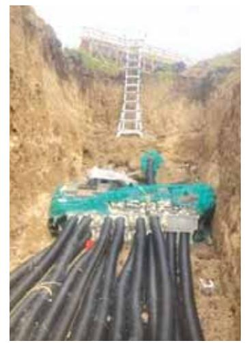
Pipes and concrete block manifold in trench.
