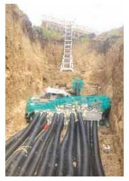
Pipes and concrete block manifold in trench.
