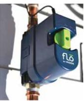
Water usage monitor senses water usage, water flow over time and total gallons that pass through the system. It has high, medium and low sensitivity settings. If a selected setting is exceeded, the valve closes, and water is shut off.
