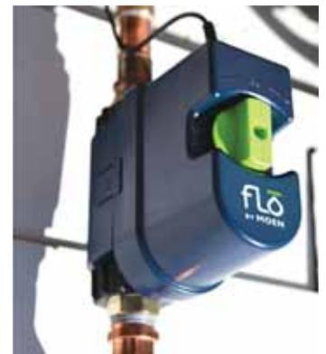
**Water usage monitor senses water usage, water flow over time and total gallons that pass through the system. It has high, medium and low sensitivity settings. If a selected setting is exceeded, the valve closes, and water is shut off.**
