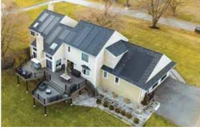
Solar shingles are designed for easy installation by roofers with a nail gun, just like regular asphalt shingles.
