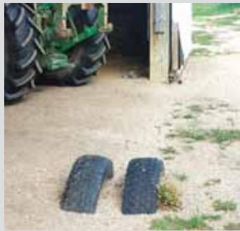
**Fritz Groszkruger, Dumont, Iowa:** "The sliding doors on my pole barn used to be held in the center by a buried post with a welded piece that fit between the rails. It didn't hold up, so I came up with the idea of using a pair of buried truck tires, spaced so the doors slide between them. Works much better.
