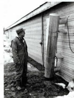
Dehumidifier is made of 8-in. dia. horizontal pipe, 10-in. dia. vertical pipe.
