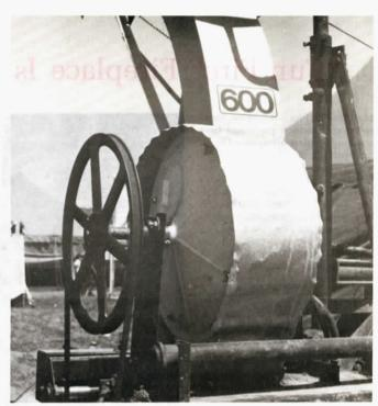
This prototype Spencer Dispenser was mounted on forage chopper to apply bloat-preventative to green chop alfalfa.
