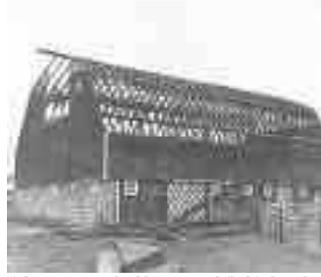
After removal of barn roof (left), local carpenters easily install new clear span roof.
