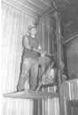
on. It slides up and down on a frame made from two 15-ft. lengths of T-beam secured to the wall. Angle iron is fitted to the inside of the T-beam flanges to serve as a track for the lift to ride in. Two sealed ball bearings mount underneath the platform on either side to run in the angle iron, while two more sealed ball bearings mount on top to run on the back side of the T-beams.
