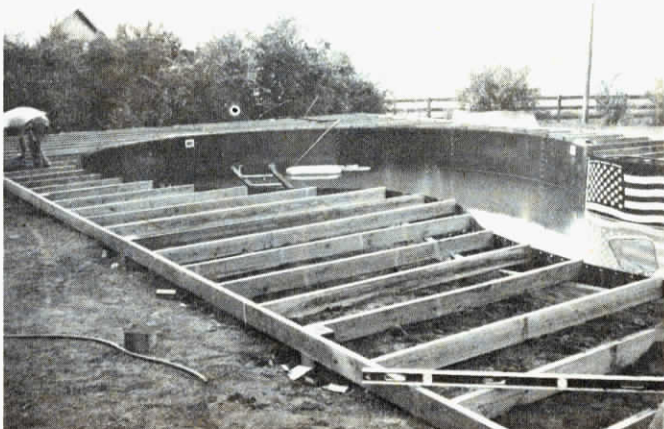
A 60-ft. long wood deck surrounds the pool, which holds 50,000 gal. of water.
