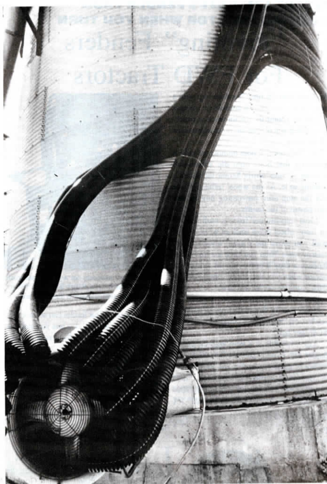
Tom Culp attaches black drainage pipe to side of grain bin.
