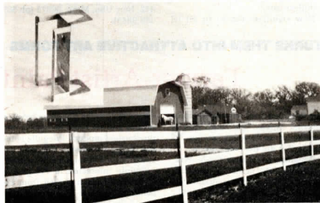
Bracket, upper left, lets you fasten wood rails to steel posts.
