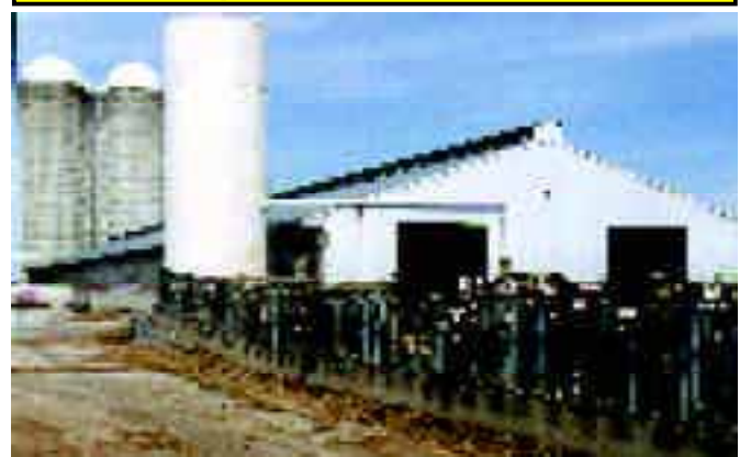
Water squeezed out by separator is returned to the lagoon. There, a pump delivers some of the water to a vertical steel flush tank at end of barn.
