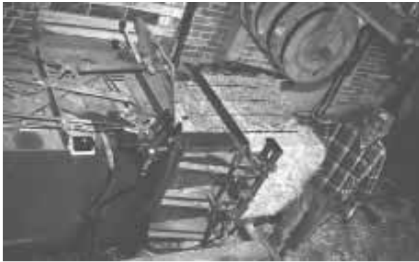
Compressed bales are bound with steel straps on drum above machine.
