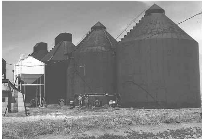
David and Martin Ray made their own bins from scratch by welding sheets of 10 and 12 ga. steel together so that they’re smooth inside and out.
