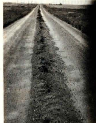
Road reworking is a 3-step process. First, a grader piles loose gravel and vegetation in the center of the road, left. Next (right) the Ridge Kicker is pulled over the pile, raking through it and throwing weeds out on top to dry. A day later, you pull through again with the Ridge Kicker set at its lowest point, which breaks up all clods and evens out the road.
