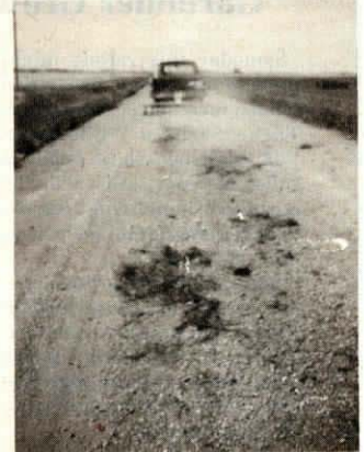
Road reworking is a 3-step process. First, a grader piles loose gravel and vegetation in the center of the road, left. Next (right) the Ridge Kicker is pulled over the pile, raking through it and throwing weeds out on top to dry. A day later, you pull through again with the Ridge Kicker set at its lowest point, which breaks up all clods and evens out the road.
