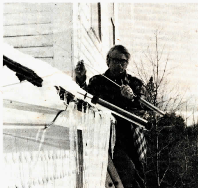
Ice lance melts a small corridor through dams at the edge of shingled roofs.
