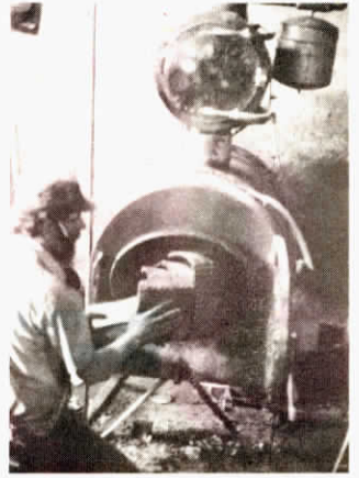
Hoppe modified Aqua Therm water-jacketed wood burning furnace by mounting afterburner on top to eliminate excess tire smoke.
