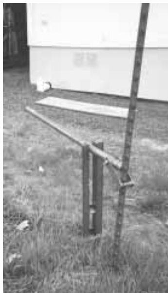
Jack is designed to stay parallel to post so post is pulled out straight.
