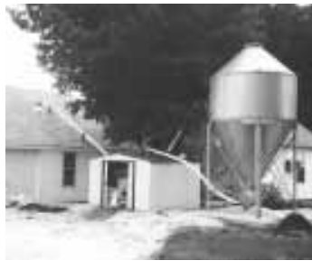
Corn is augered from bulk bins to corn burner that heats house and office.
