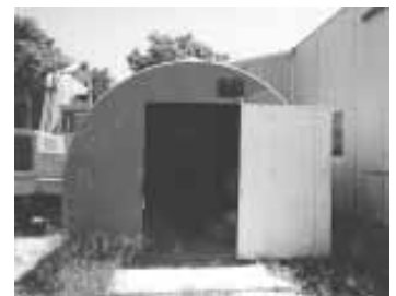
Shed is made from 15,000-gal. diesel tank.
