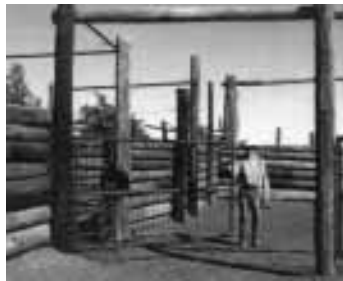
Poles are stacked on top of each other to make sides.
