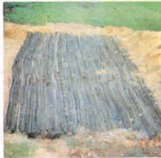
Gillmore's making a "rubber driveway" using strips of tire tread nailed together.
