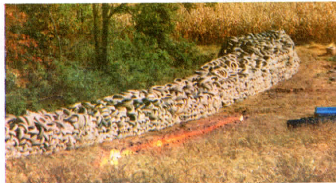
Photo shows a portion of Boohar's deer fence which is made up of 200,000 tires.
