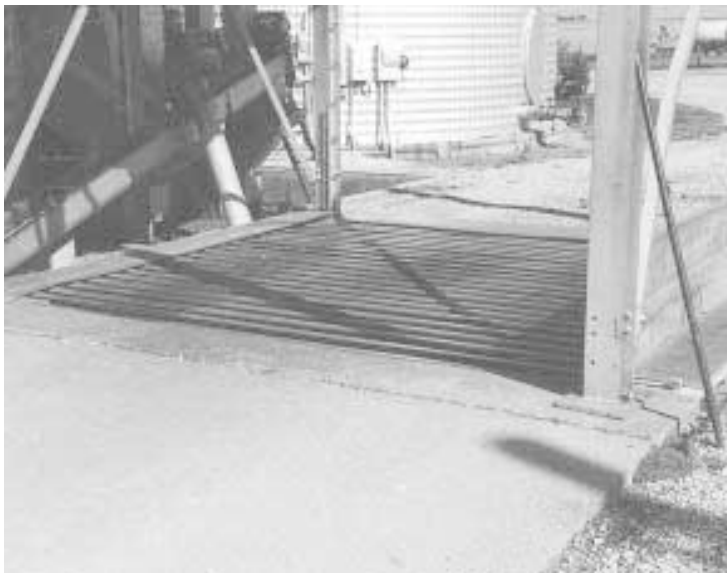
Home-built pit holds 500 bu. and is covered by 10-ft. long railroad rails.
