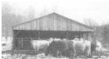
Open side of shed faces south and serves as a shelter for calves born in spring.
