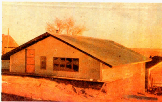
Sod building is topped by wood-frame construction, anchored by a 4-in. thick concrete slab laid atop the building's 5-ft. thick walls.
