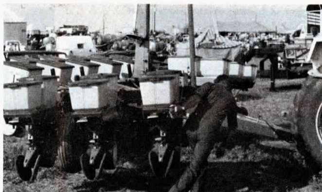
Kelderman "hinged" 12 row Deere planter folds to 16 ft. road width in minutes.
