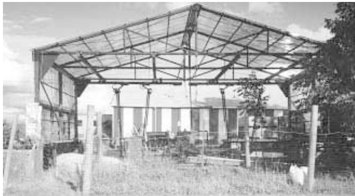
Photo shows a small version of “rolling greenhouse”. Vandendorre built another one that’s 240 ft. long by 40 ft. wide.
