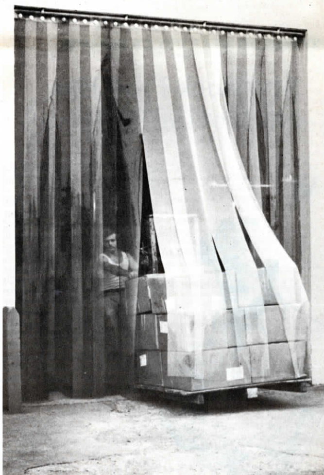
Clear vinyl strips can be hung to provide from 50 to 100% overlap of the individual strips, depending on how "weathertight" a seal is desired. The percent overlap also governs noise-dampening effect of the strip door.
