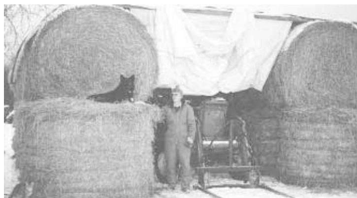
Walls of the “shed” were made by standing bales on end and then placing a second layer on top setting crosswise.
