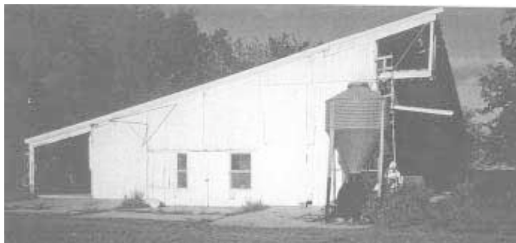
Barn roof slopes from 8 ft. on lower end to 22 ft. on upper end. South-facing fiberglass panels let in heat and light.
