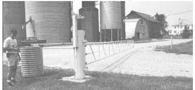
Imhoff’s 45-ft. gate is powered by a 1/2 hp Craftsman garage door opener.
