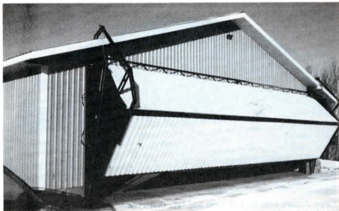
As a pair of hydraulic cylinders are extended, the two halves of the door are raised and "sandwiched" together horizontally, leaving the entire door opening clear.
