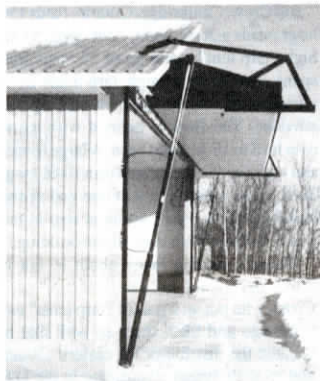
A pair of hydraulic cylinders run from the ground up to the door's framework.
